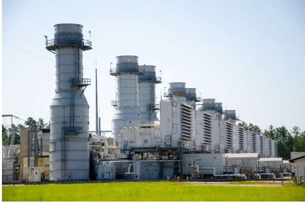
Peaking Facility near Sandersville, Georgia
